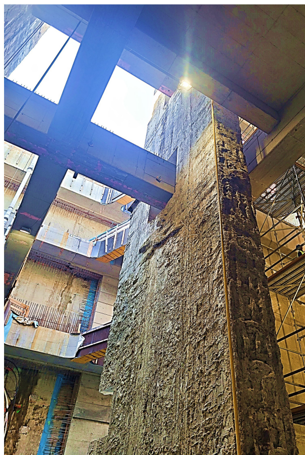
Figure 2. Reinforced concrete structures of the metro line under construction (photo by Julian Sigmund (TU Wien), 2023).
