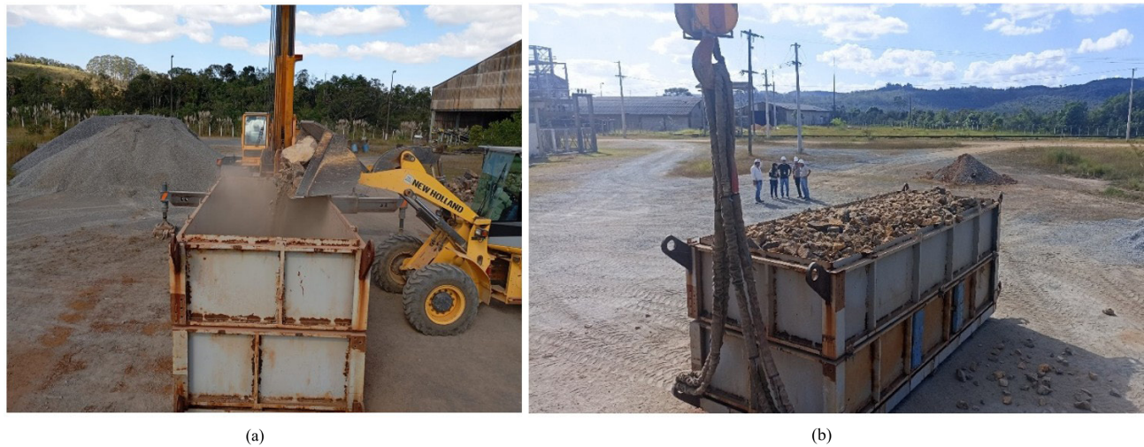
Figure 4. Filling the shear box with the rockfill material: (a) filling in progress; (b) filling completed.
