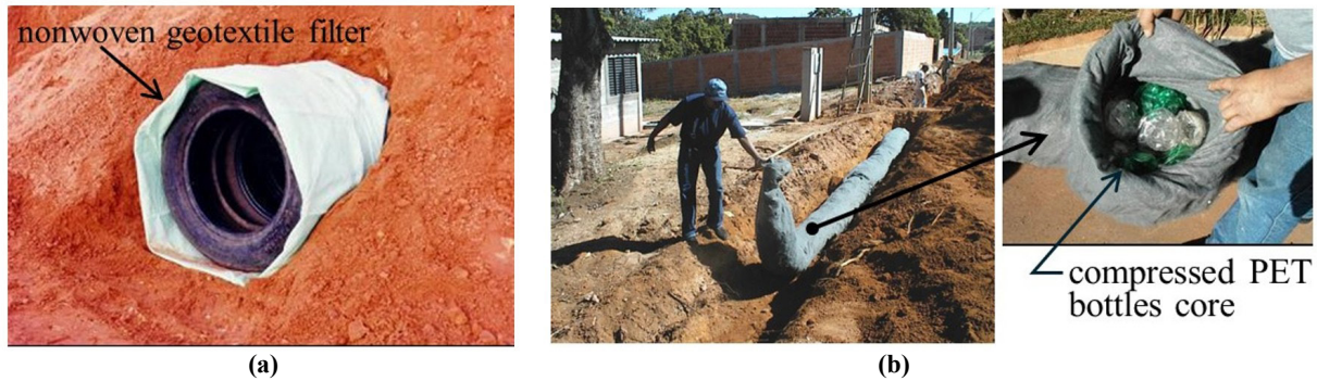
Figure 27. Combination of geotextile filter with alternative drainage materials: (a) geotextile and scrap tires in a landfill; (b) geotextile and compressed PET bottles in an urban street.
