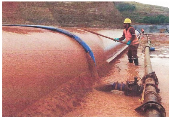
Figure 18. Geomattress during the dewatering process at Risoleta Neves dam site (courtesy Dr. A.R.S. Fahel).
