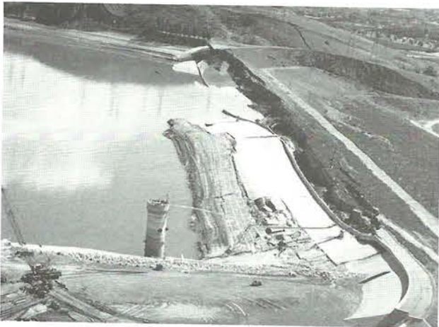
Figure 4 - Lower S. Fernando Dam failure.
