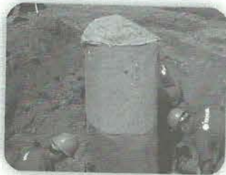
Ringtrac® Ring reinforcement for granular columns on soil improvement
