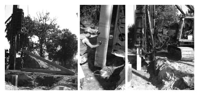
Figure 4 - Sequence of the execution tasks for the precast concrete driven piles.
