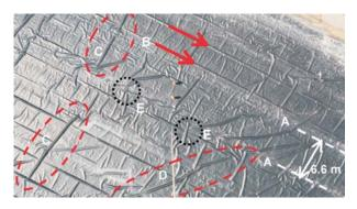
**Figure 7** - Air photo of geomembrane installation. 1.5 mm smooth HDPE; Camera elevation 65 m; Latitude 43 °16' N; Air temperature 28 °C; 1:20 pm Aug 18 2006 (modified from Chappel *et al.* 2007).
