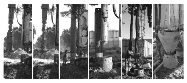
Figure 5 - Sequence of the execution tasks for the bored piles with temporary casing.
