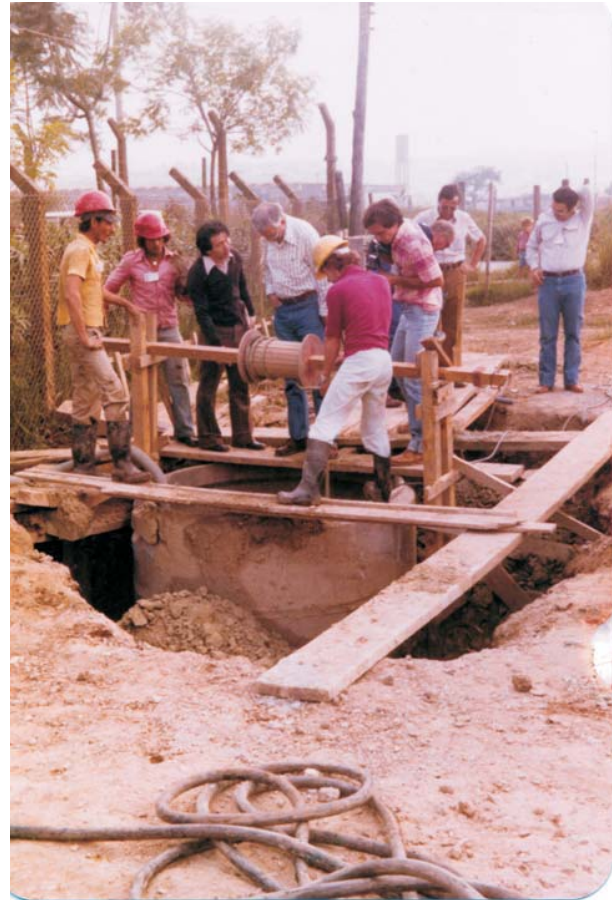
Figure 11 - Trial shaft for the River Tietê tunnel.
