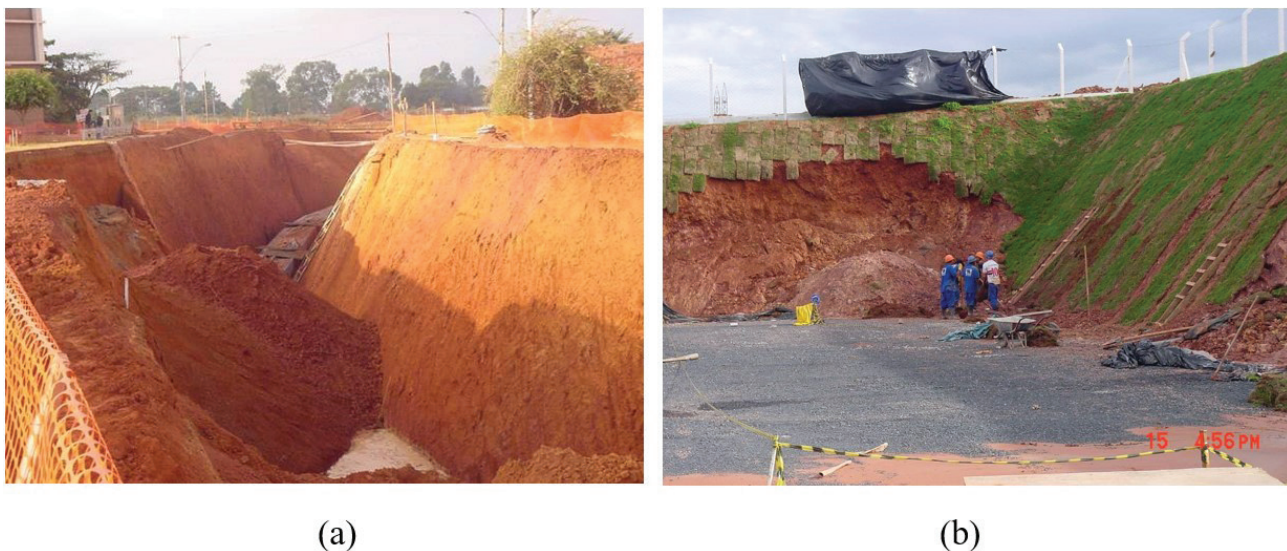
Figure 30. Slope failures in excavations (Camapum de Carvalho et al., 2007).
