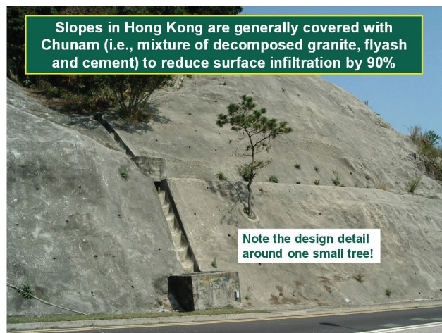
Figure 9. Use of chunam in Hong Kong to maintain the stability of slopes.
