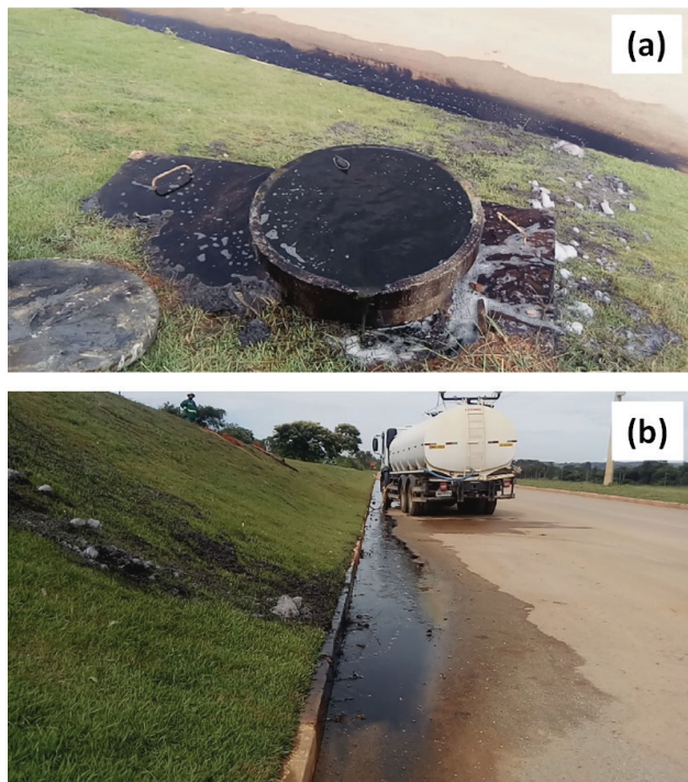
Figure 4. Leachate leaks: (a) gas drainage with leachate; (b) flow of leachate along the road.
