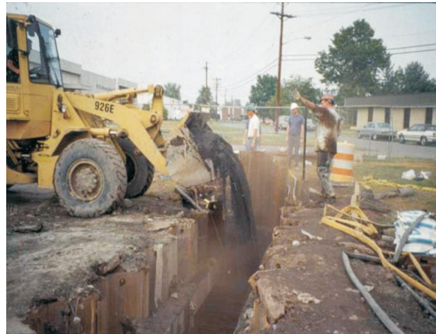
Figure 15. Filling of a supported trench with a mixture containing ZVI (zero-valent iron) for building a continuous-trench PRB (From ITRC, 2011).
