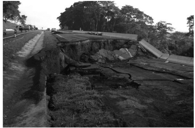
Figure 15. Geotechnical failure of the northbound lane of SP-334.
