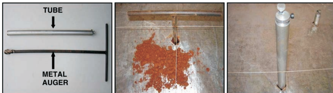
Figure 11 - Installation of monitoring tubes.
