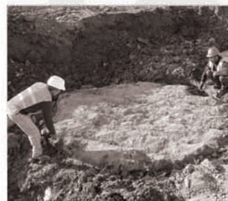
Grouting Jet Grouting Compensation Grouting
