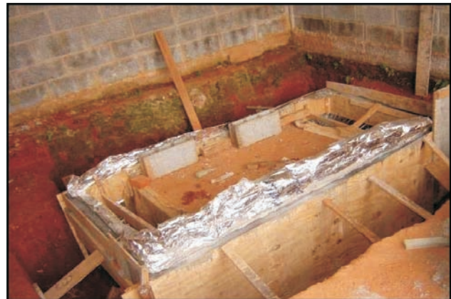
Figure 7 - Side cement walls.
