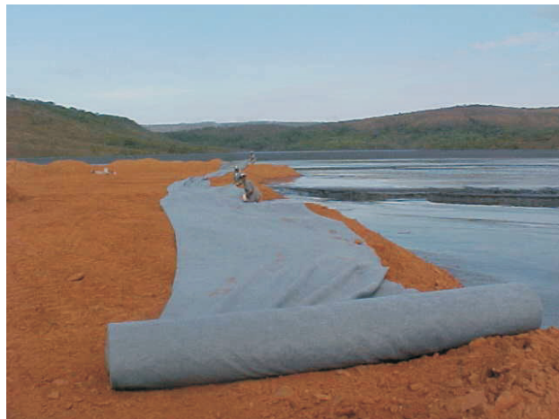
Figure 15 - Placing the geosynthetic on the tailings.
