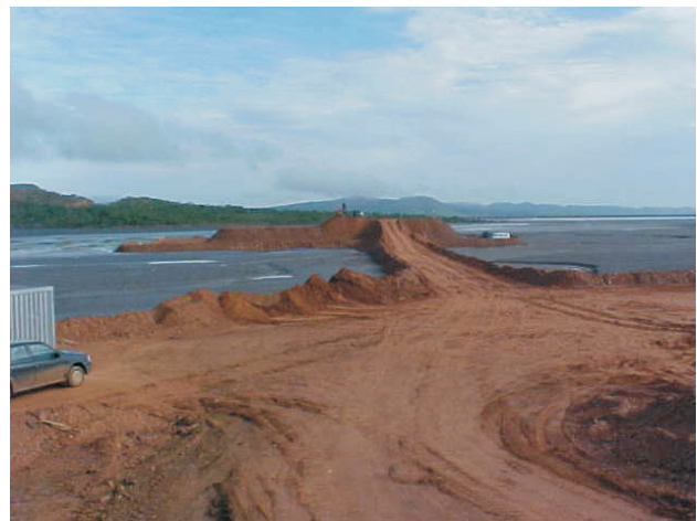
Figure 4 - Embankment at 5 m height.
