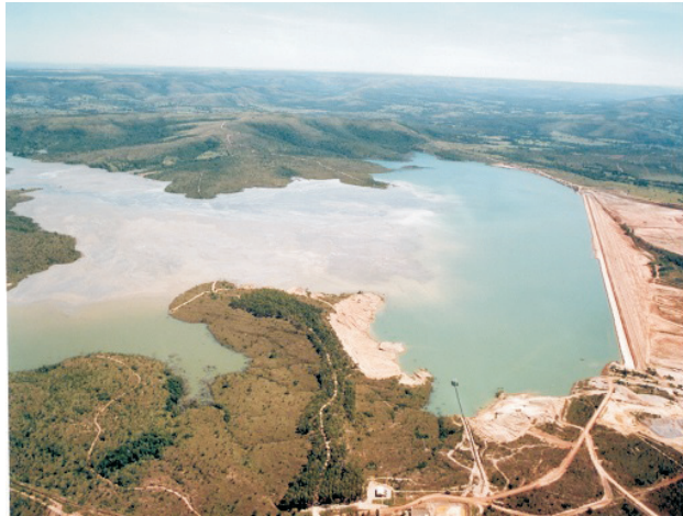
Figure 1 - Morro do Ouro tailings dam.
