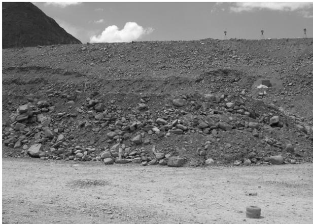
**Figure 3** - Caracoles dam under construction (2007). San Juan, Argentina. Detail of the gravel fill.
