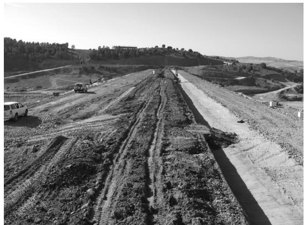
**Figure 6** - Lechago dam. Core, filters and rockfill shoulders.
