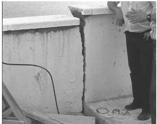
**Figure 10** - Collapse settlements of rockfill in Calanda dam.
