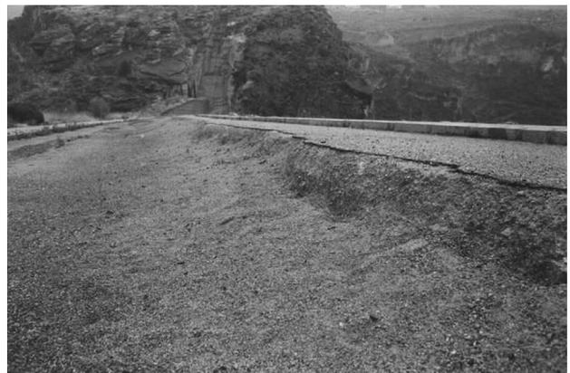
**Figure 11** - Collapse settlements of rockfill in Martín Gonzalo dam, Córdoba, Spain.
