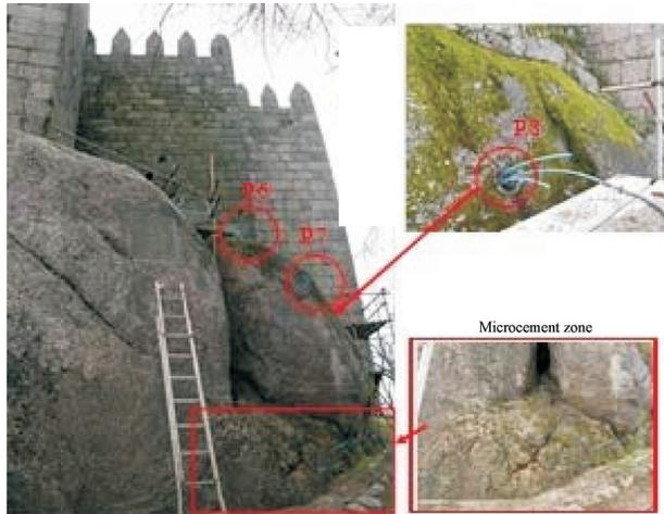
**Figure 24** - Arrangement of nailings and consolidation zone with micro-cement.
