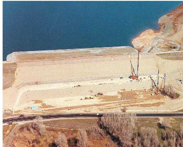
**Figure 13** - Installation of stone columns and gravel mini-column drains beneath the downstream embankment of Mormon Island Auxiliary Dam in 1994. Note the excavation and steepened slope needed for development of a working platform and for optimization of the improvement zone location for its effectiveness as a key block.
