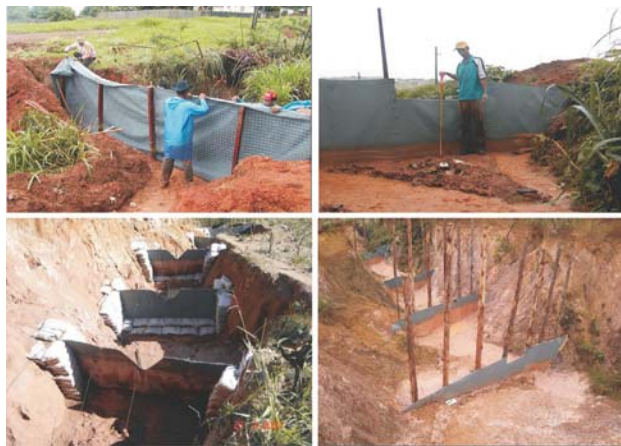
Figure 37 - Examples of a low cost erosion control solution involving the use of geotextiles (Courtesy of Dr. Rideci J. Farias and Furnas Centrais Eléctricas).
