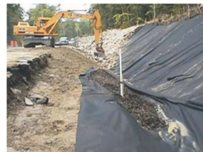
c) Geotextile filter combined with tire chips.
