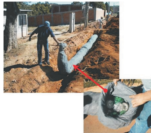
a) Geotextile filter combined with compressed PET bottles.
