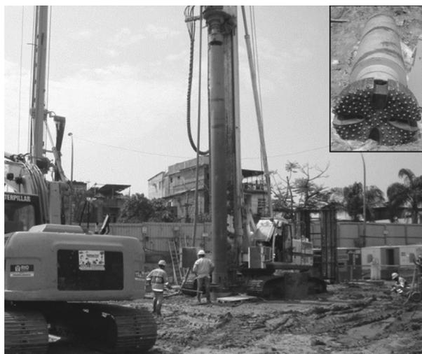
**Figure 7** - Equipment used to drive (by turning and pushing down) a steel casing, diameter 80 cm, and then lower a DTH hammer, 70 cm diameter.
