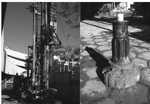
**Figure 6** - Equipment used to drive (by turning and pushing down) a steel casing, diameter 50 cm, and then lower a DTH hammer, 39 cm diameter.
