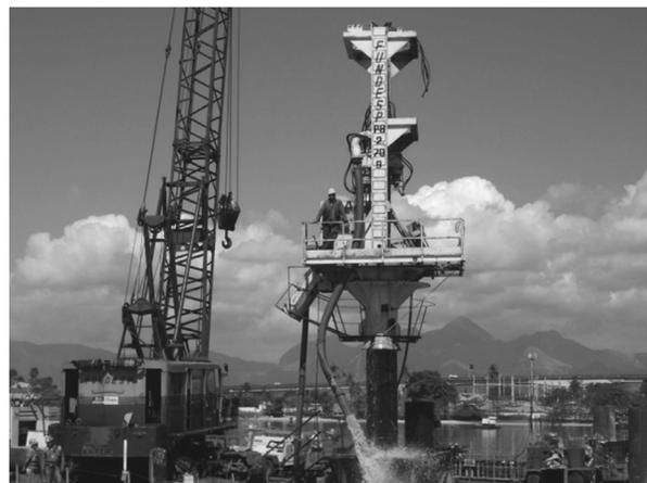
**Figure 5** - Rotary equipment for rock drilling, with rock bit diameter 70 cm, sitting on top of an already impact driven steel casing, diameter 80 cm.
