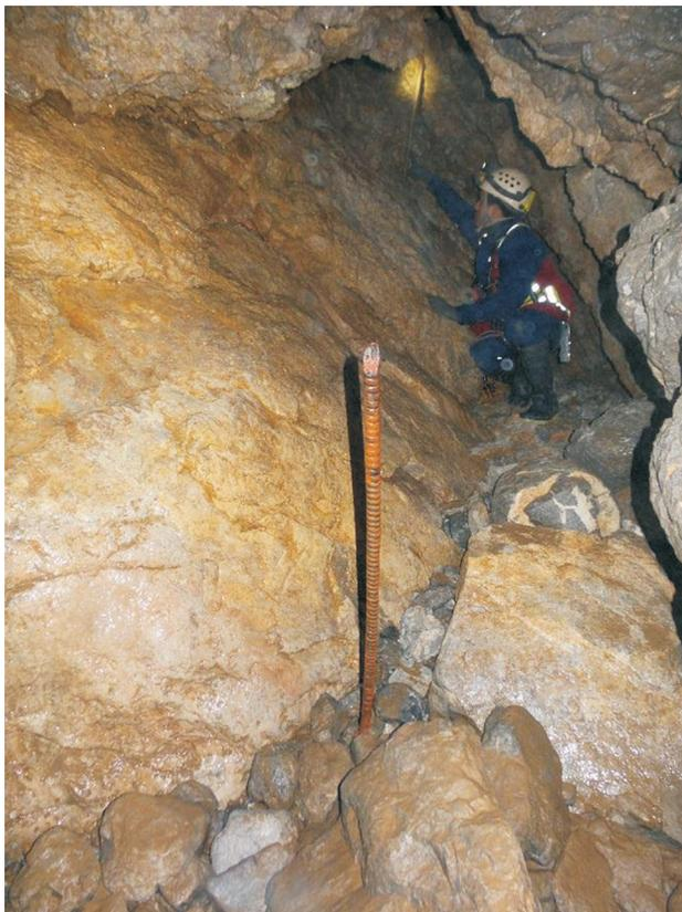
**Figure 68** - View of a headrace tunnel rock bolt. The fact that the bolt is vertical suggests that the area being inspected is above the roof of the tunnel.
