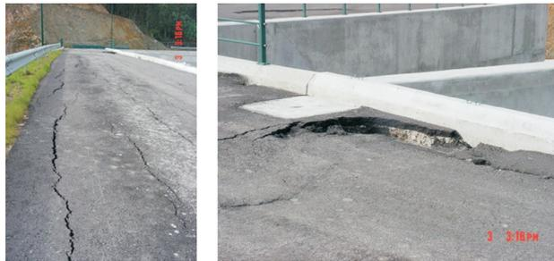
**Figure 22** - Extensive cracking and settlements at the crest.
