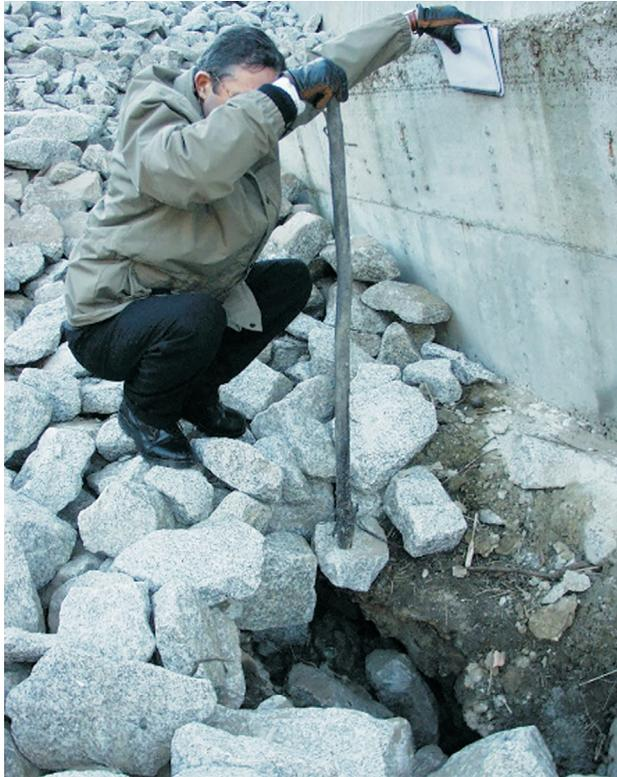
**Figure 27** - Upstream sinkhole in the spillway vicinity.
