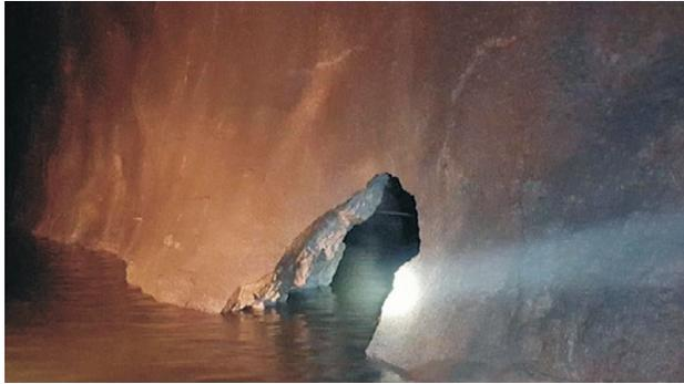
**Figure 67** - View of the entrance to the cavity on the hydraulic left sidewall of the headrace tunnel at chainage 12+740.
