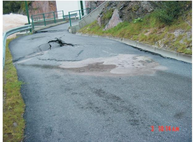
**Figure 24** - Sinkhole in the access to the bottom outlet valve.
