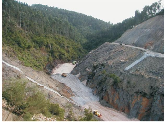
**Figure 21** - General view of the bottom valley before construction and during the placement of the drainage blanket.
