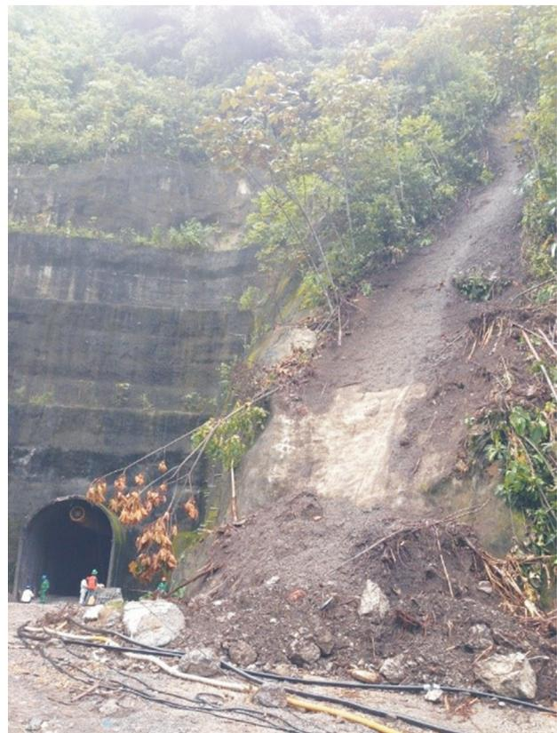
**Figure 63** - Adit 2 – landslide near the entrance portal.
