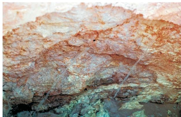
**Figure 7** - Canaliculi at Balbina hydroelectric power plant dam foundations.
