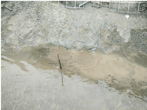
**Figure 42** - Soil boiling at the slope toe (Caldeira *et al.*, 2017b).
