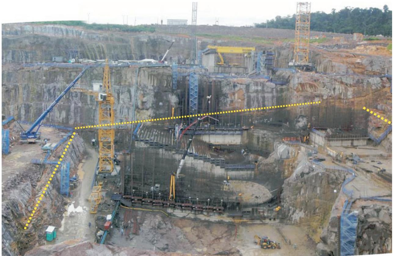
Figure 32 - Master joint trace emphasized in yellow, as visible at the excavation walls.
