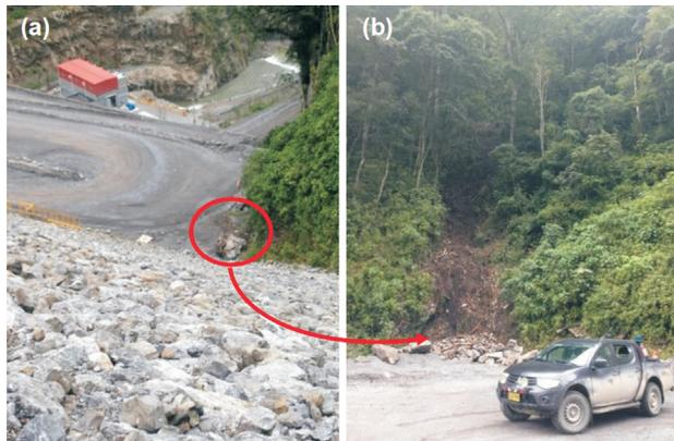
**Figure 62** - Right bank – landslide downstream of the dam.
