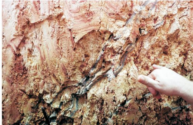
Figure 16 - Inspection trench – clacage planes intersecting and treating canaliculi.
