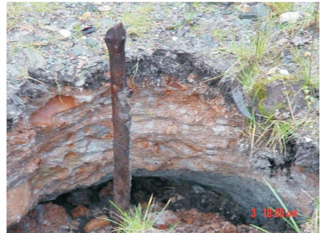
**Figure 23** - Sinkhole in the berm over the toe drain.
