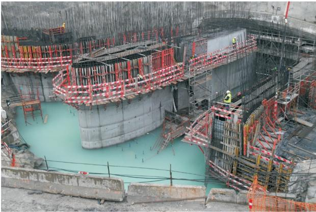
**Figure 41** - Inundation of the cofferdam interior up to elevation 138.0 m in November 2016 (Caldeira *et al.*, 2017a).
