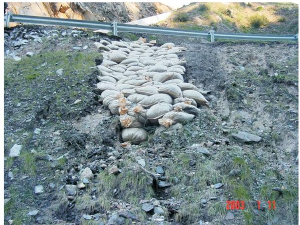
**Figure 25** - Sand bags placed inside the sinkholes.
