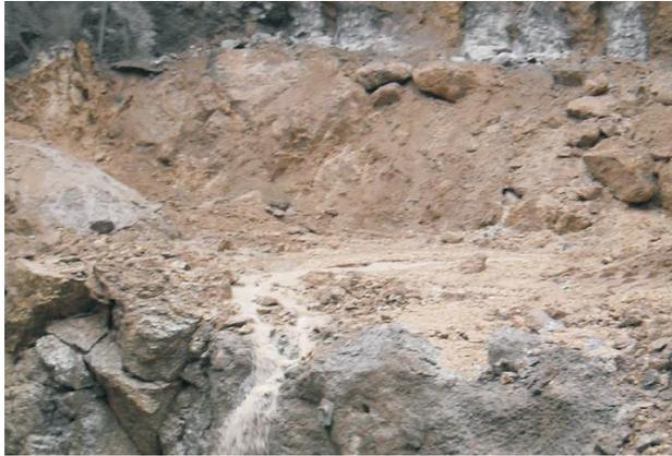
**Figure 40** - Exit point of the flow with the formation of a pipe and fines entrainment (Caldeira *et al.*, 2016b).
