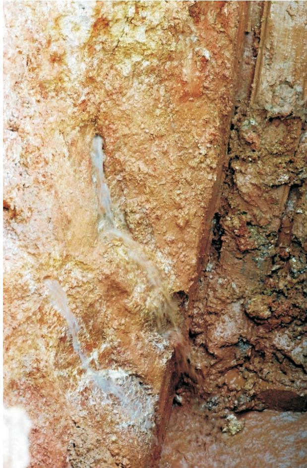
**Figure 8** - Canaliculi at Balbina hydroelectric power plant dam foundations.
